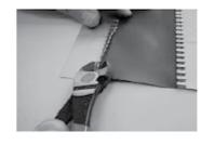
Lift the seam outward to a right angle.
